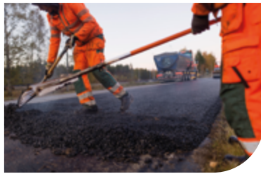
Construction materials and asphalt
