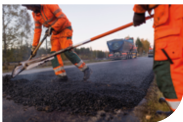
Construction materials and asphalt
