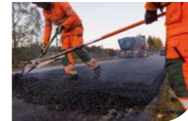
Construction materials and asphalt
